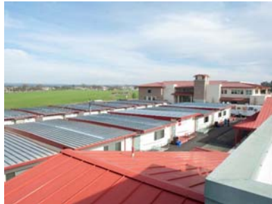
North County Interim Housing Completed Summer 2015
