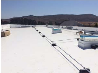
1000s Complex Roofing/HVAC Completed Summer 2019
