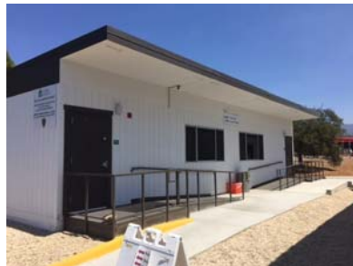
San Luis Obispo Interim Housing Phase I Completed Summer 2015
