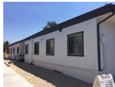
San Luis Obispo Interim Housing Phase II Completed Spring 2016
