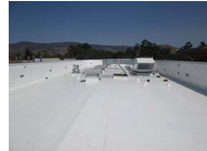
San Luis Obispo Roofing/HVAC Upgrades Completed Winter 2016/2017
