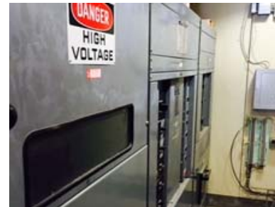
San Luis Obispo Main Campus & 1000s/2000s Electrical Switchgear Replacement Completion Winter 2019
